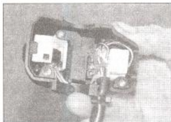
21.5c . . . then inspect the wiring connections and switch contacts
