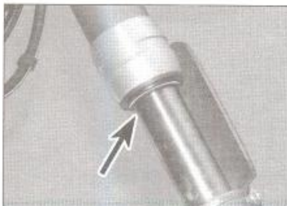
25.3a Check for signs of grease or oil leaks . . .
