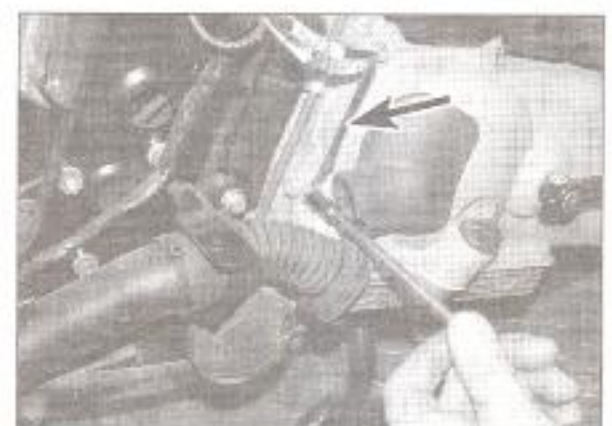
5.8b . . . and the engine earth wire (arrowed)
